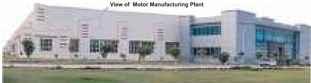
View of Motor Manufacturing Plant
