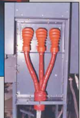
Raychem's cold applied boots installed in Ring Main Unit (R-Cab)
