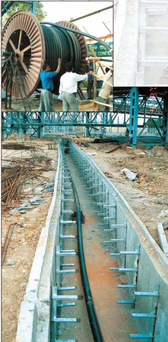
EHV 132kV cable installation work
