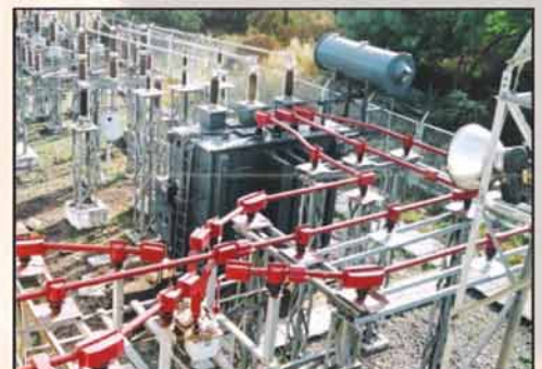
Insulation of Switchyard with BBIT, BPTM, HVBT and BCIS components
