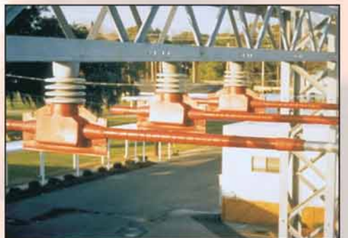
Insulation of Switchyard with BBIT, BPTM, HVBT and BCIS components
