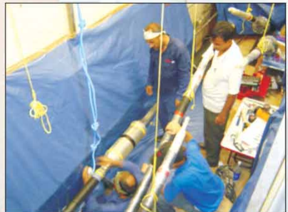
Installation of EHV cable joints
