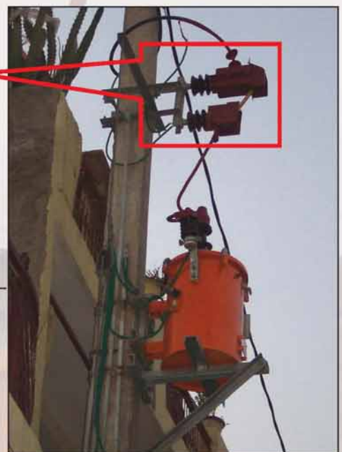
D.O fuse after insulation
